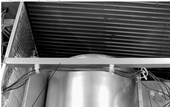
FIGURE 5 HEATER KIT INSTALLATION
